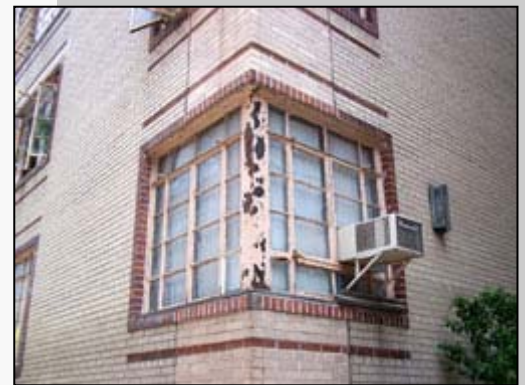
Rare steel frame window still intact though in need of maintenance at 101 Cooper Street.
