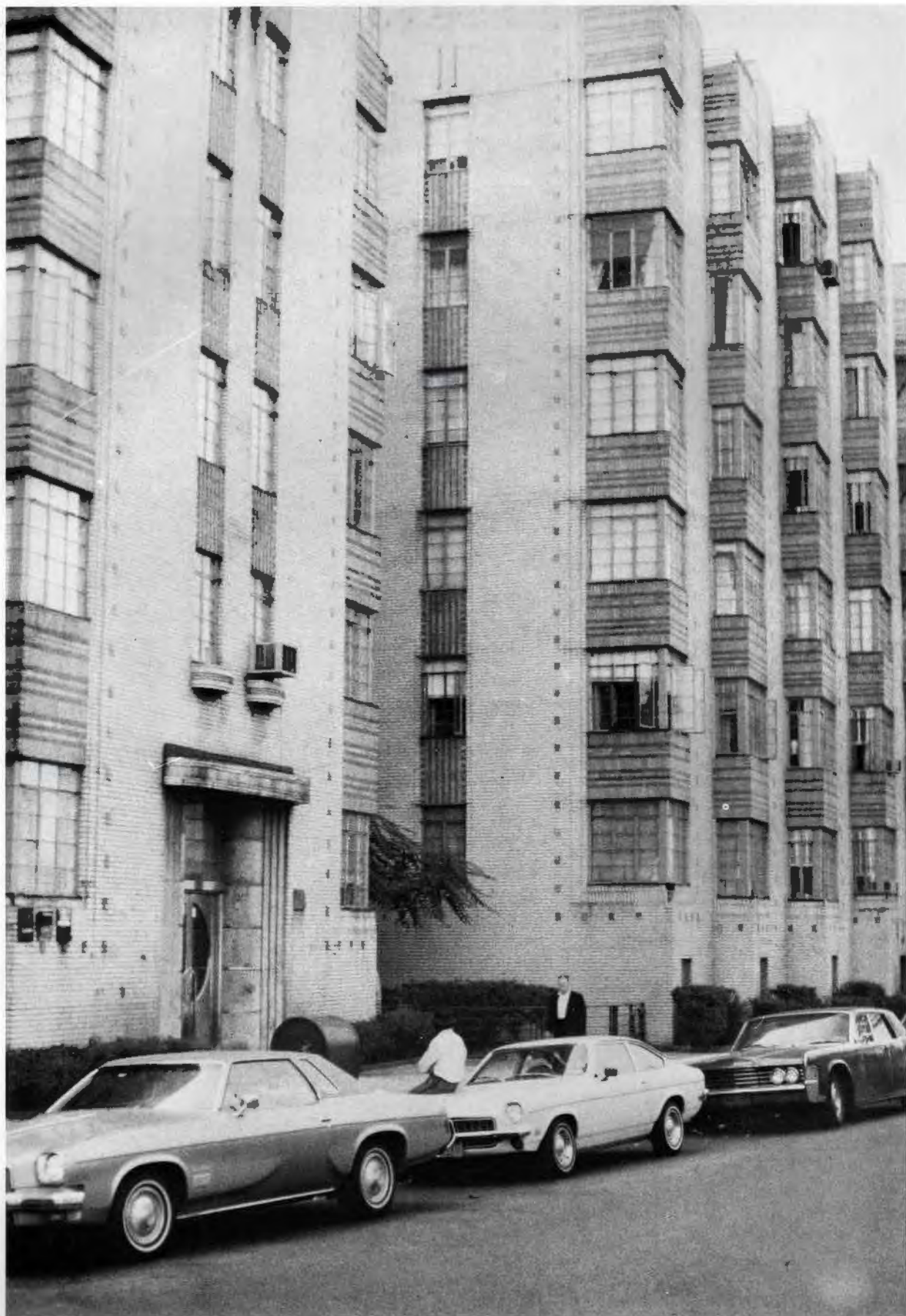
Grand Concourse streetscape.
